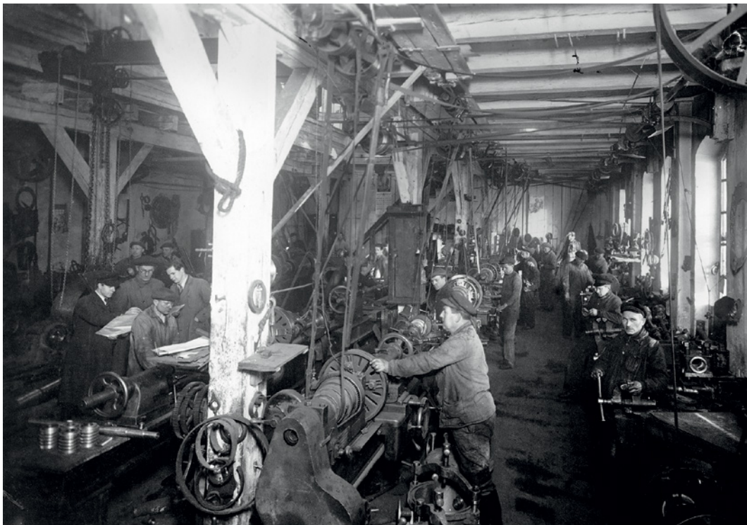
Mechanical work benches in the factory at the beginning of the 20th century.
