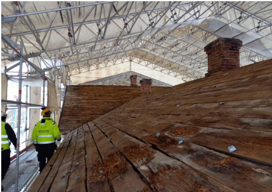
Fig. 4.3. Old school roof renovation for weather protection at Padasjoki, 10/2020.
