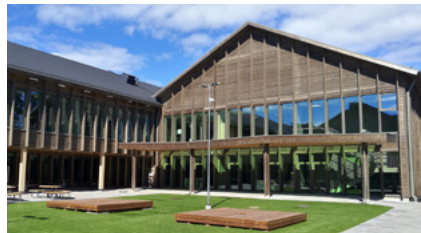
Fig. 5.1. Dry chain construction under the tent (Saari, 2019).
