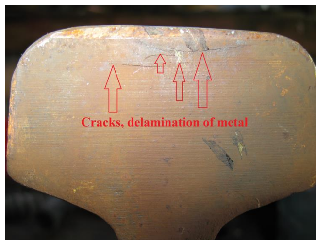
Fig. 3.5. Defect with code X10.1 found in railroad section Vecumnieki–Lāčplēsis.
