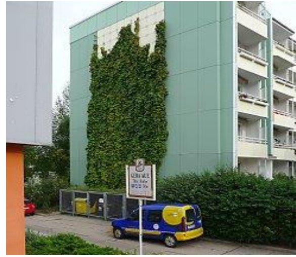
Fig. 1.14. Green wall formed by Dutchman's Pipe in the large-scale housing estate in Erfuhrt-north, Germany [225].
