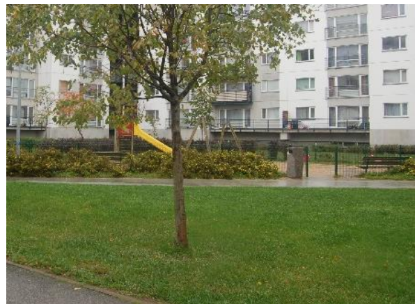
Fig. 2.7. Children playground in the area of new social housing Raadiku, Tallinn, October 2018.
