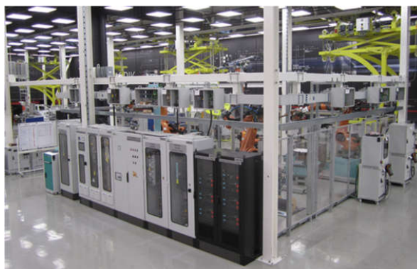
Fig. 2: DC microgrid realization as automotive manufacturing cell for experimental analysis.
