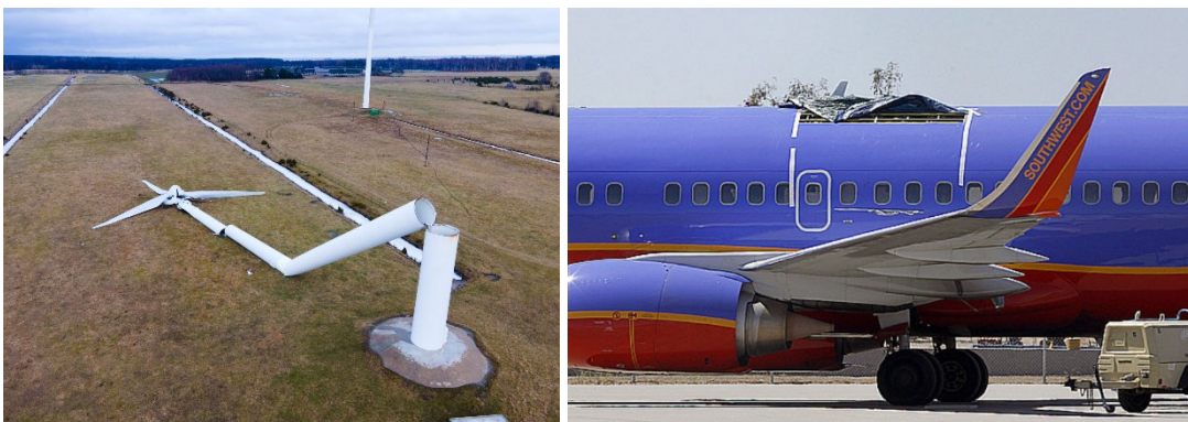
Fig. 1. Major structural failures. Left: Saaremaa, Estonia 2022; right: Yuma, Arizona 2011.
