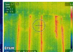
Figure 7. Tower floor in the attic.
