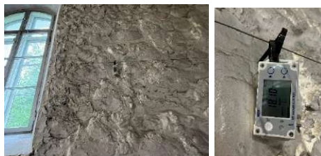
Figure 2. Example of mounting HOBO MX measuring instruments on the outer wall.
