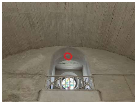
Figure 3. Example of mounting HOBO MX measuring instruments on the ceiling arch.
