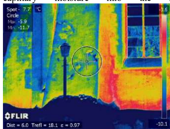
Figure 4. Wall of Cesis Church from outside
